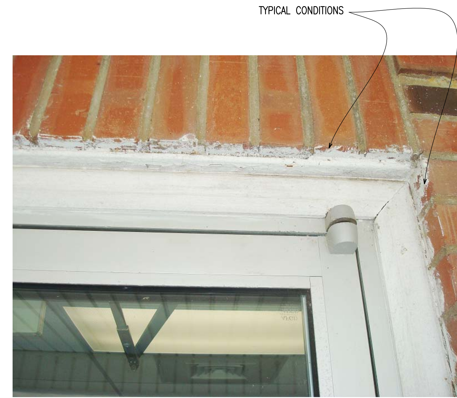
3 PHOTOGRAPH A-201A-901 EXISTING BRICK SURFACE N.T.S.
