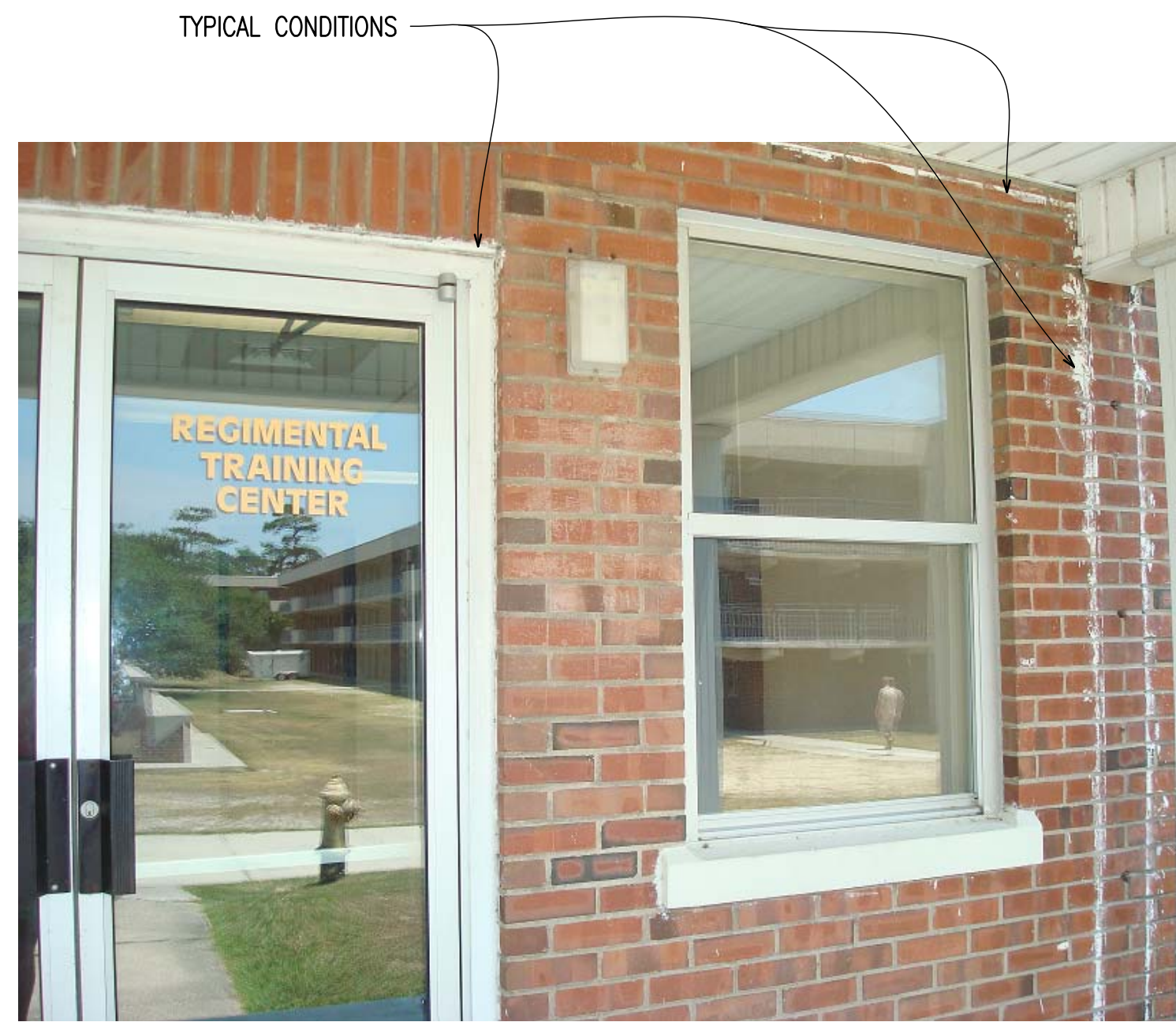
1 PHOTOGRAPH A-201A-901 EXISTING BRICK SURFACE N.T.S.
