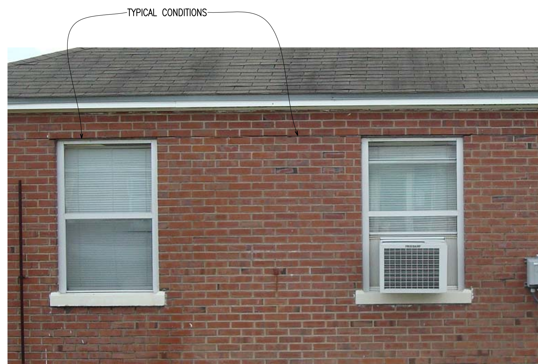
9 PHOTOGRAPH A-201A-901 EXISTING EXTERIOR BRICK N.T.S.
