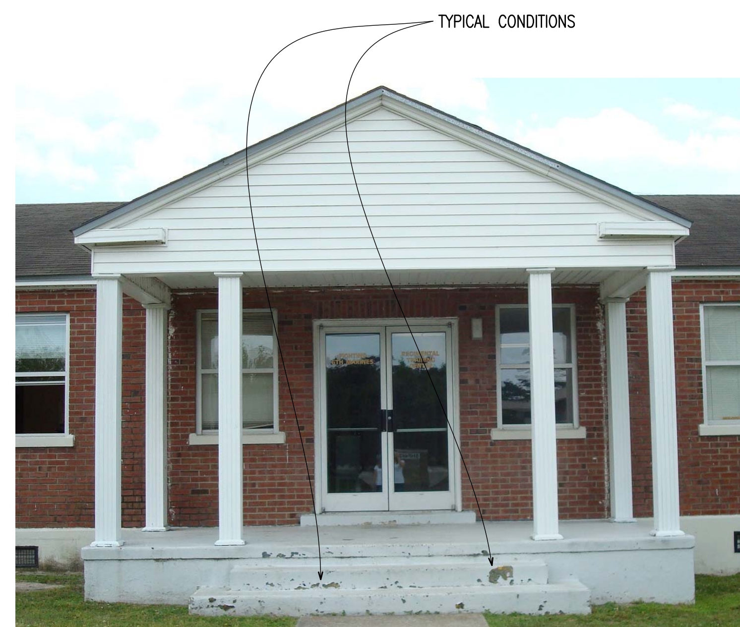
6 PHOTOGRAPH A-201A-901 EXISTING FRONT PORCH N.T.S.
