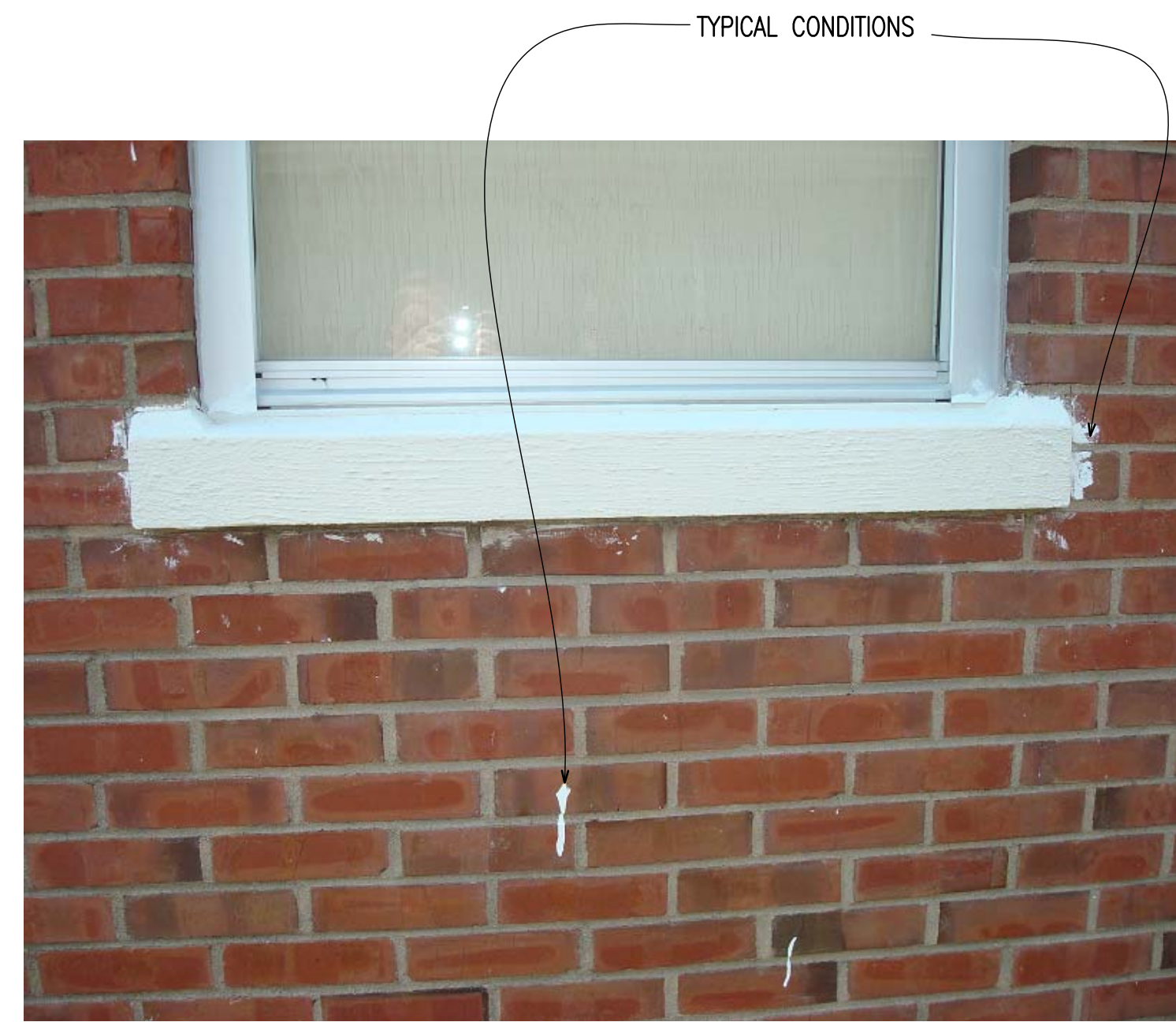
2 PHOTOGRAPH A-201A-901 EXISTING BRICK SURFACE N.T.S.
