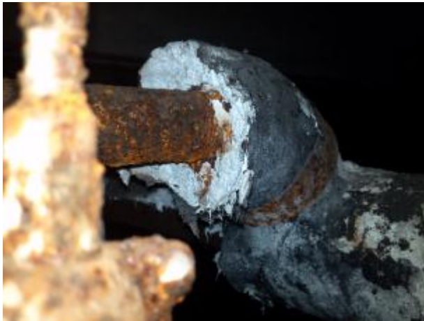
HA-1 and 2: Thermal System Insulation
