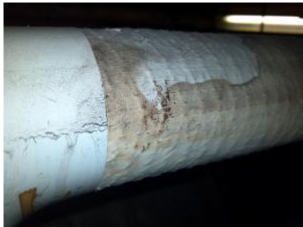
HA-6, 10, 15 and 18: Mastic Coating on Thermal Pipe Jacket Cover
