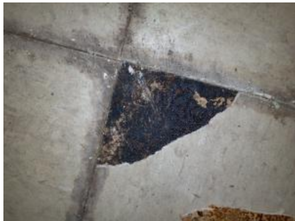
HA-4, 8, 14, 17: Mastic Associated with Floor Tile
