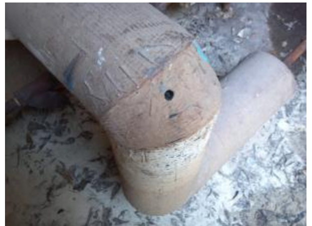
HA-9 Black Sulfur and Glass Insulation
