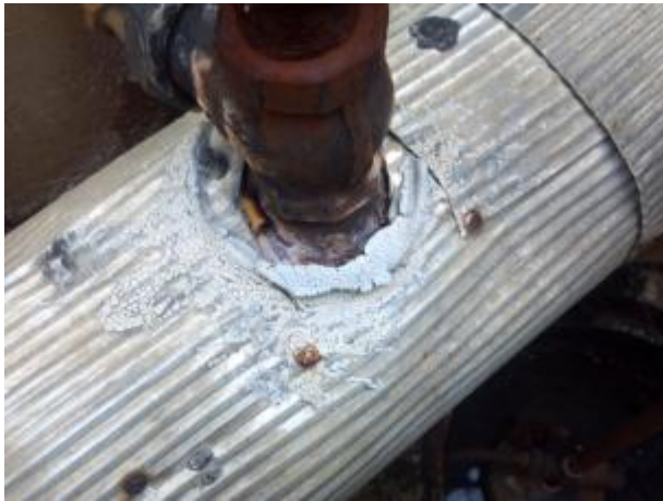
HA-11 and 12: Caulking on thermal Pipe Wrap
