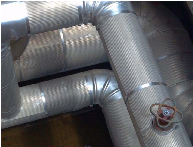
Silver Pipe Casing (Photo 03)
