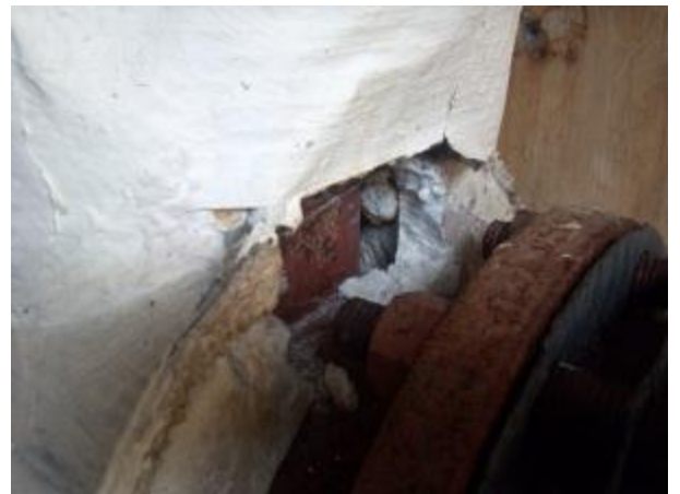
HA-5: Pipe Insulation
