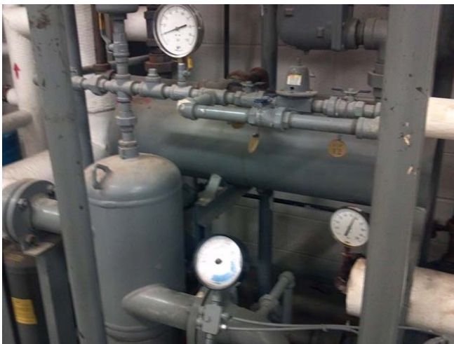
Gray in color Tank Boiler (Photo 03)
