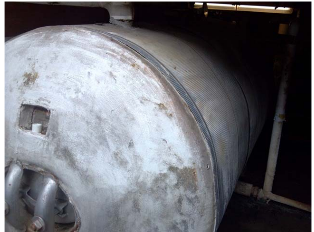
HAs-2,4,5,6,9,11,15,17,18,20: Tank Insulation
