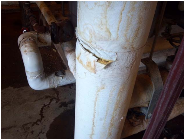
HAs-1,13,23: Mastic Coating on Thermal Pipe Insulation
