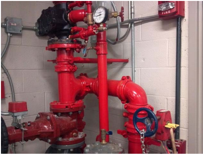
Red in color interior Riser (Photo 01)
