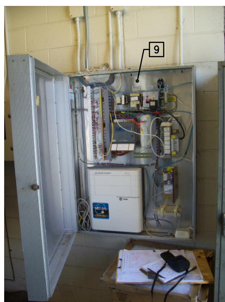
PHOTO 7 EXISTING DDC CONTROL PANEL
