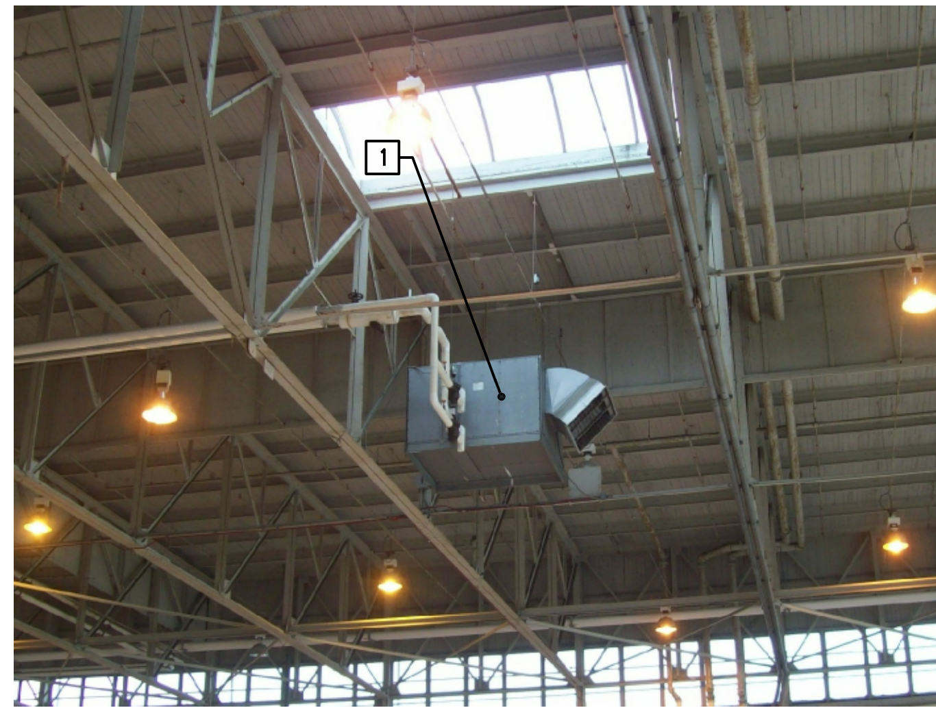
PHOTO 8 EXISTING HEATING/VENTILATING UNIT
