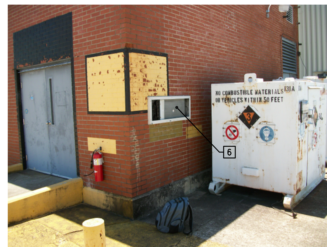
PHOTO 5 - BUILDING 131 NORTH EAST CORNER
