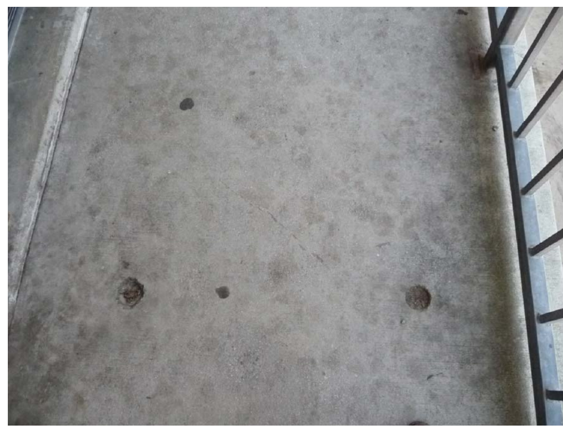
1 TYPICAL SPALLING CONCRETE REPAIR 24 LOCATIONS AT \pm 2\frac{1}{2} " DIAMETER X \pm \frac{1}{2} " DEEP N.T.S.
