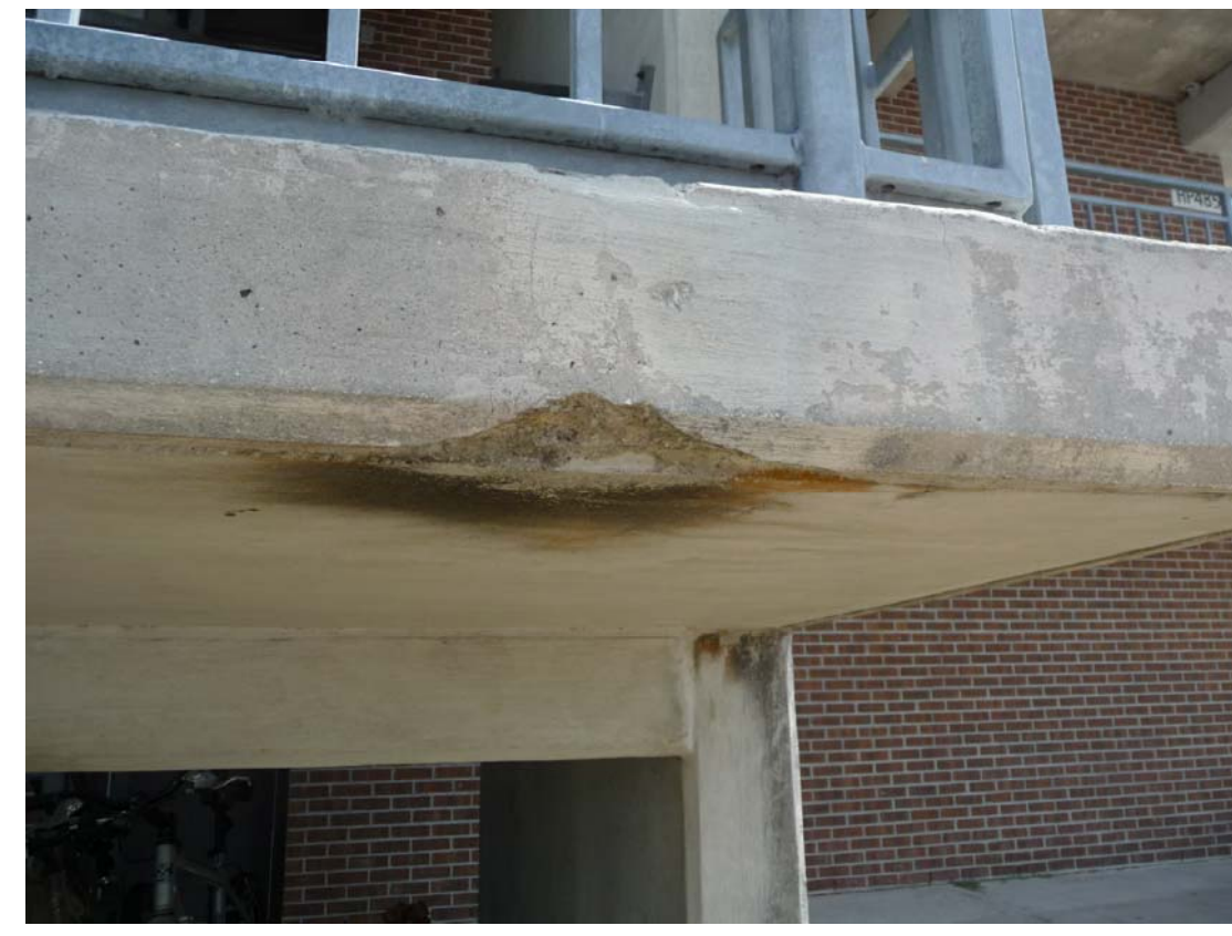
3 TYPICAL SPALLING CONCRETE REPAIR 30 LOCATIONS AT \pm 4 " DIAMETER X \pm 1 " DEEP N.T.S.
