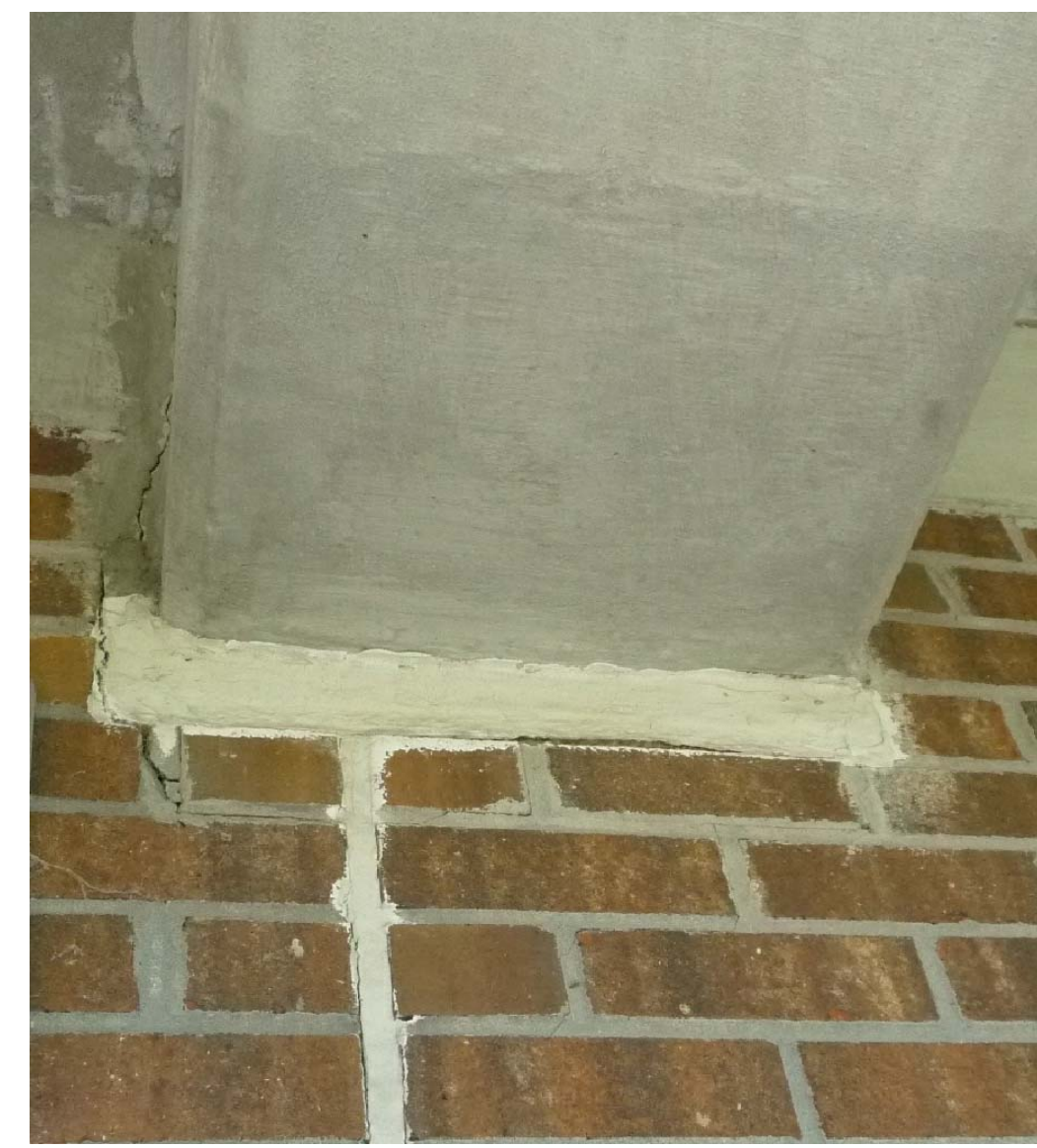
5 TYPICAL CRACKED MASONRY REPAIR 2 LOCATIONS AT \pm 12 " IN LENGTH N.T.S.
