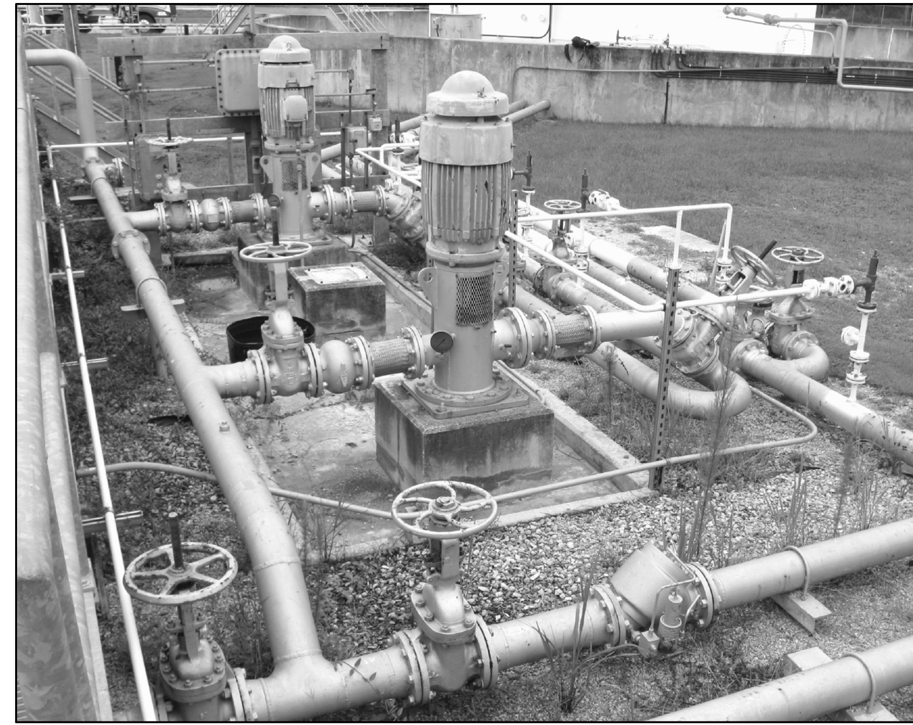
PUMP PAD, NORTHERN PORTION D3 MD401
