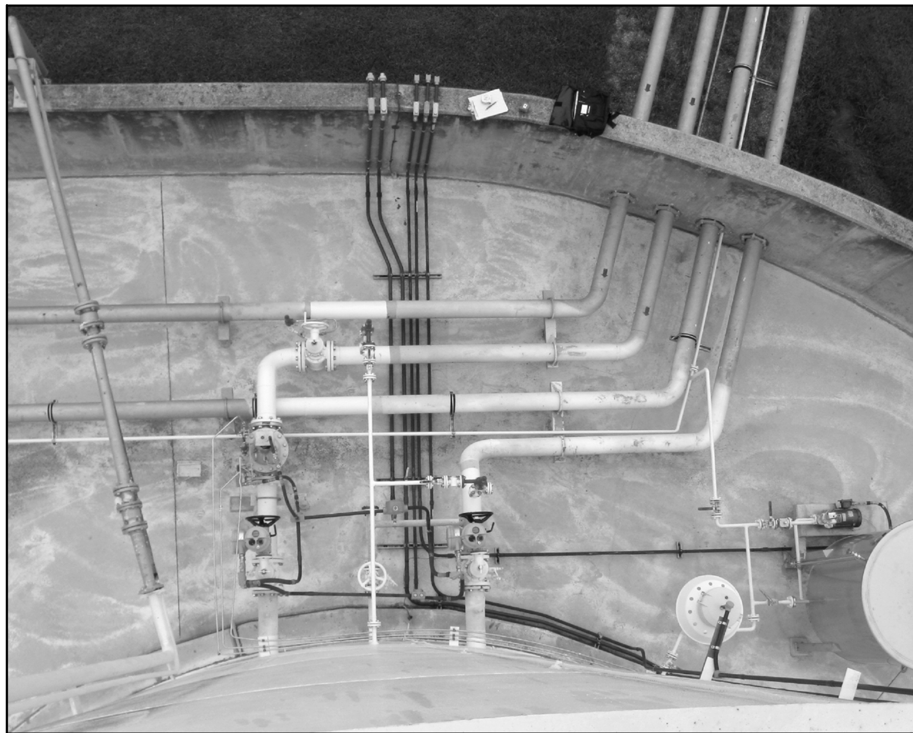
TANK 3 PIPING D4 MD401
